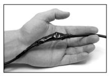
After taping the wire ends individually, wrap the entire connection with electrical tape as shown. This will help protect from moisture and prevent the wires from breaking contact.
